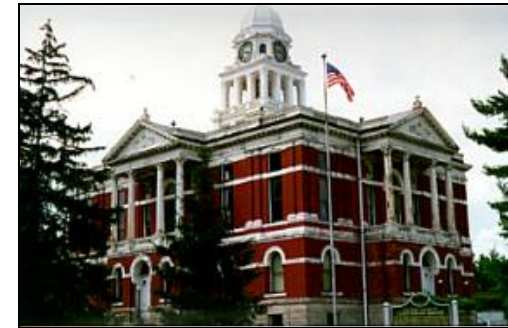
Second County Courthouse-Built 1883-86
