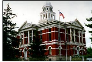
Second County Courthouse Built 1888
