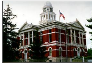
Second County Courthouse Built 1888
