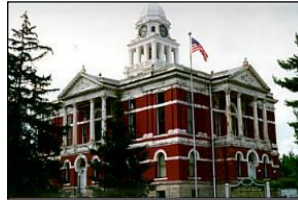
Second County Courthouse Built 1888
